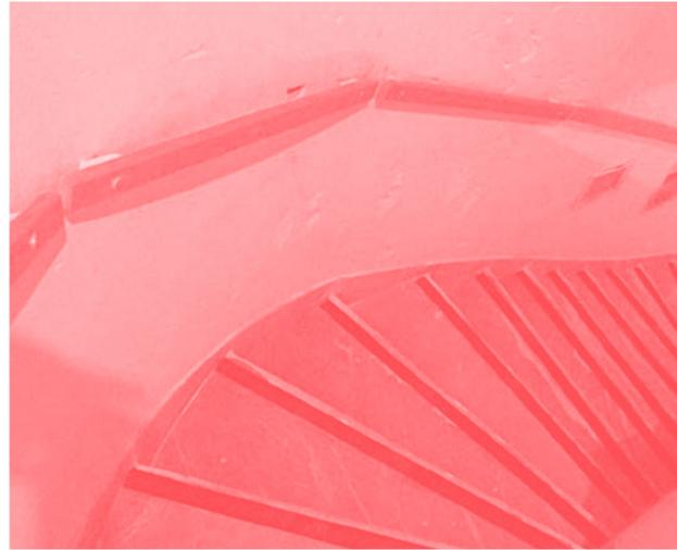
**CURRENT PHOTO 7.B.** View of the staircases, in which repairs to damaged stairs were executed and the installation of non-slip tape and wooden handrails can be observed. COMDEC June 2019
